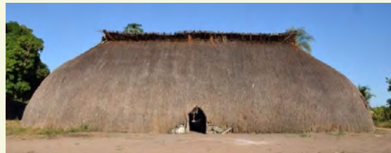
Casa Kamaiurá: “walls that breathe”, with layers of straw.
